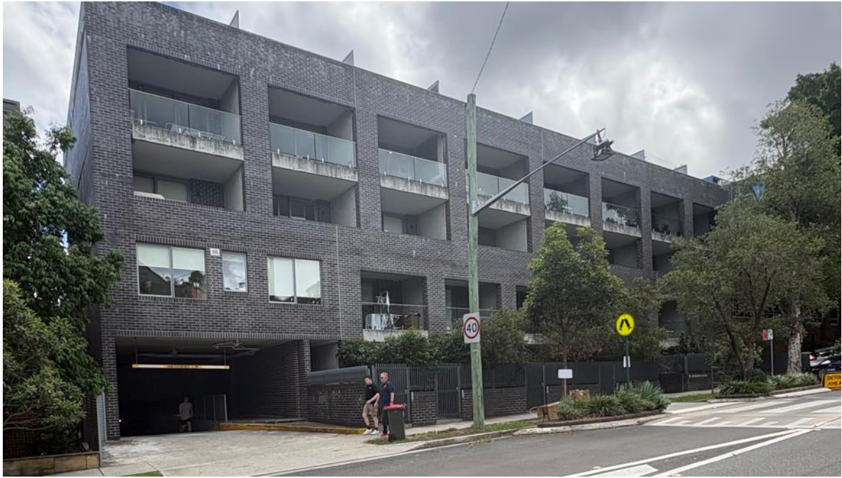
Figure 1: 12 Primrose Avenue, Rosebery, viewed from the south-east.
